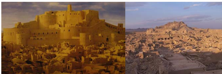
Figure 1. Bam Citadel Before & After earthquake
